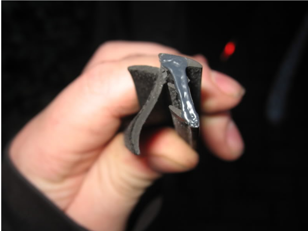
Shape of new window seal.
